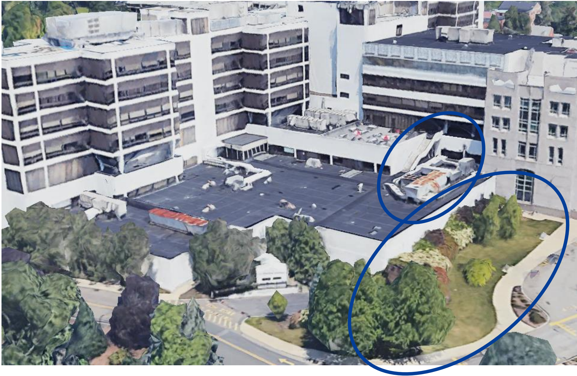
Replace Existing Roof Top Unit – January 2023/March 2023 Site Prep – November 2022/February 2023
